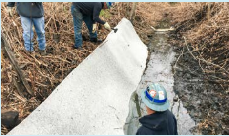
HalenHardy® crew installing Spilltration® Husky rolls to stop the erosion of a ditch leading to a trout stream.
