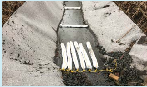
Job complete. Husky filter liners on both banks. SkimBoa oil sheen filter socks installed to capture fugitive oils.
