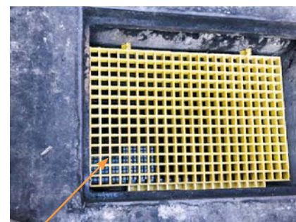
Step 2: Install Pre-Cut Fiberglass Grating
