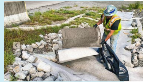
Spilltration® Husky culvert inlet filter sleeve protects trout stream from TSS & FOG. Change out monthly. NEED CUSTOM SIZES? CALL 814-822-2004.
