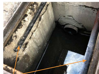
Step 1: Install L-Channel Brackets
