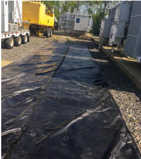
Ground Pads installed underneath the HardyBerm to protect from rock punctures.
