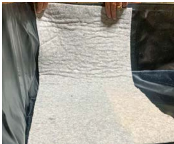
STEP 1: Cover Patent Pending Snoutlet viaduct with HuskyFlex pre-filter fabric.
