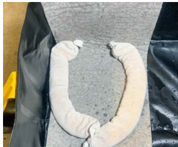
STEP 2: Clip HuskyFlex to berm wall and place SiltTrap socks on top.
