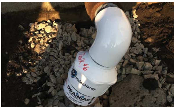
For complete drainage install Drainiac® filter as near to vertical as possible
