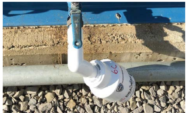
1-inch PVC Drainiac® adapter for smaller drain fittings
