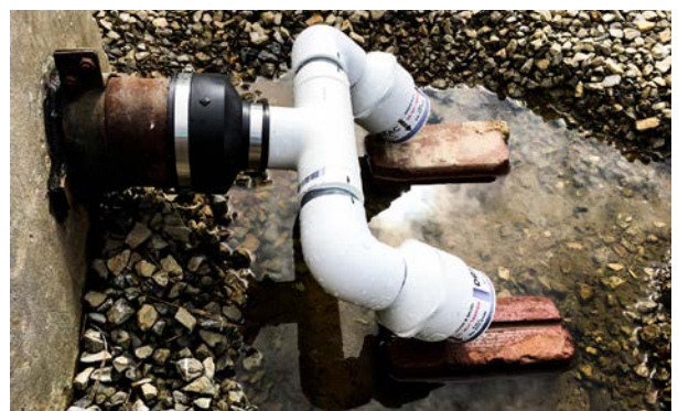
Build a manifold for faster filtration of larger containments
