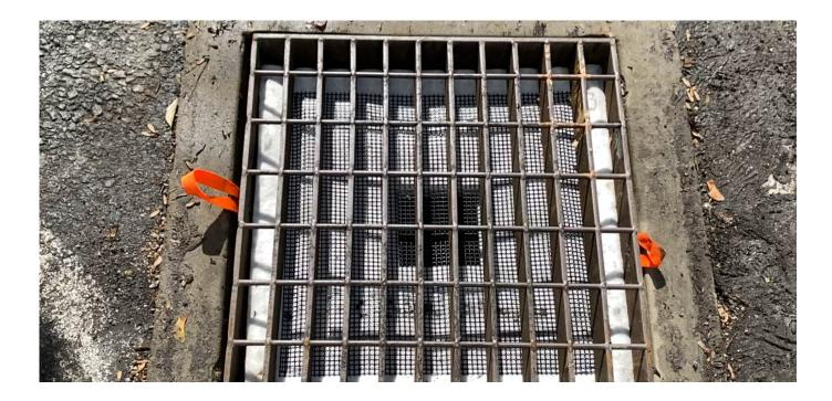
Storm drains are the last opportunity to capture silt, sediment and oil sheen before it is discharged into receiving waters.
