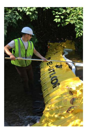
Constructing underflow dams in ditches, creeks and streams to contain and control oil or fuel spills is a proven response technique. However, it is resource intensive. When time is critical and personnel are in short supply, utilizing prefabricated underflow dams that can be deployed by two responders in less than 10 minutes can greatly affect the outcome of initial responses.
